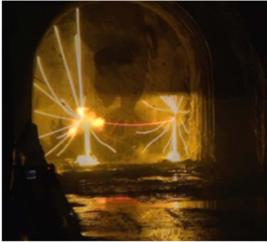
Blasting for Y-arm completion (Dec. 2013)
