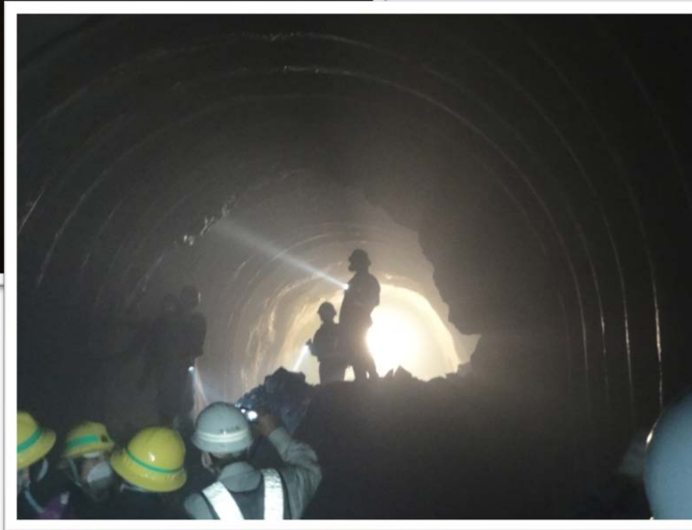
Blasting for Y-arm completion (Dec. 2013)
