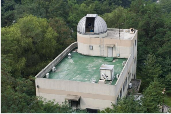
SNUO 0.6m Telescope (RC) Currently, 20' x 20' CCD 1 degree imager in future with a focal reducer
